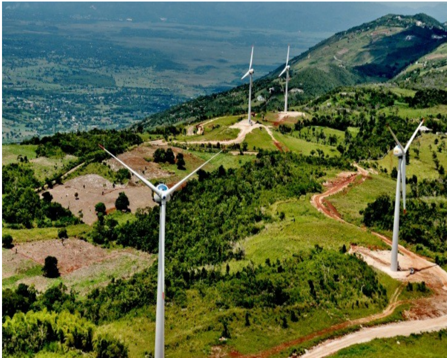
Jamaica Public Service Company Ltd
